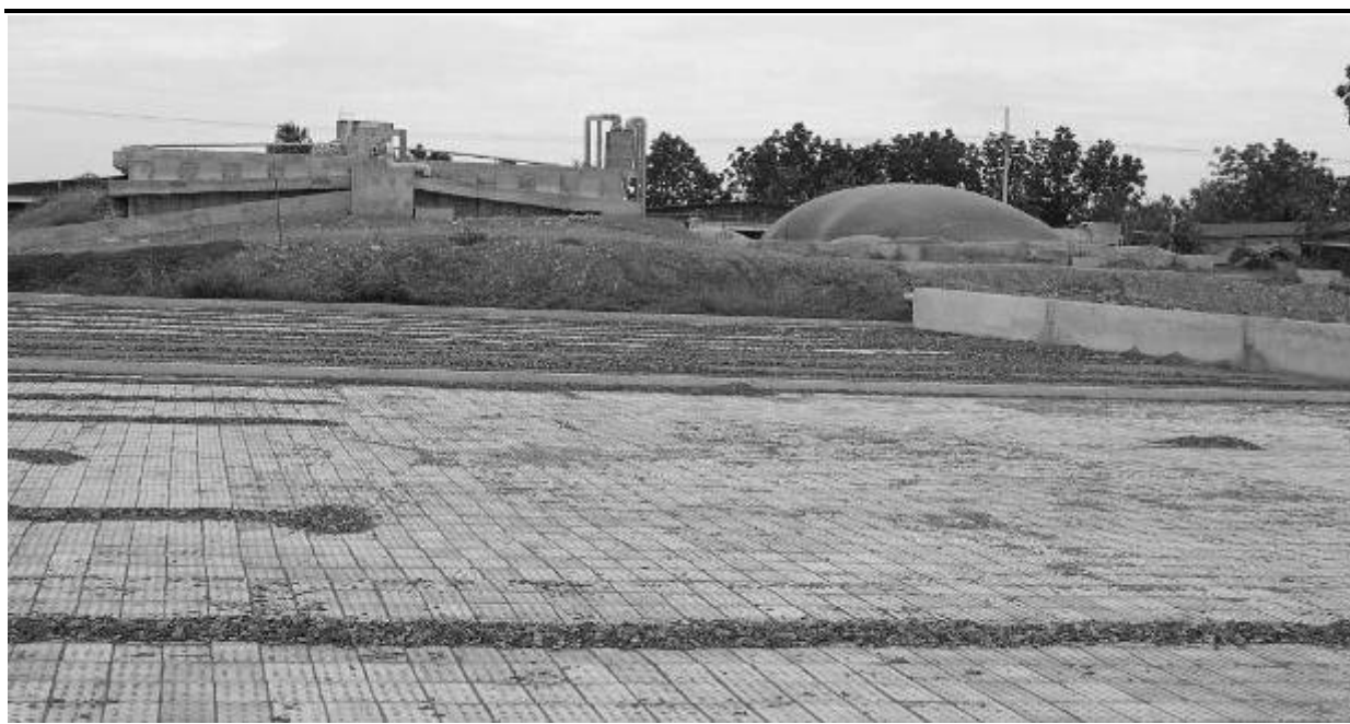
Box 2 Final effluent solids drying bed, SPM Farm
