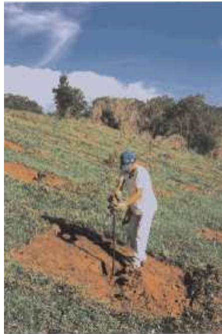
Picture 12: Making of holes and mincing. Observe the contour cleaning completely free of weeds and sods. Notice the depth of the hole and the minced soil which is reutilized for the planting process
